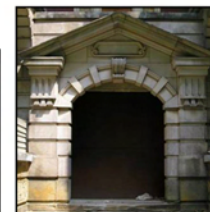
East Boulevard Apartment Pediment Entry
