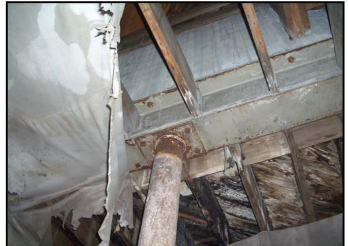
Second floor wood joist and wood sheathing has completely deteriorated.
