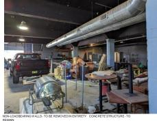
NON-LOADBEARING WALLS- TO BE REMOVED IN ENTITIETY CONCRETE ST REMAN BUILDING A - NORTH
