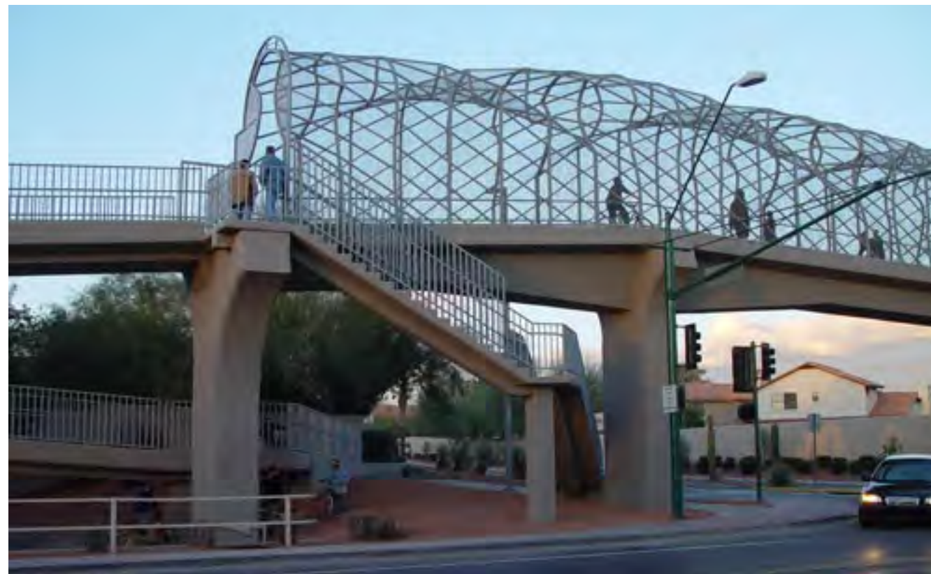
Sculptural frame covered in chain link with decorative metal railing when bridge is not over roadway
