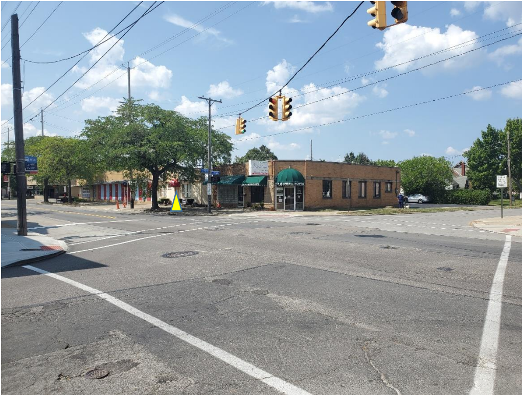
Another view of the art site. The locust tree will remain in place and not be affected by the street-reconstruction work.
