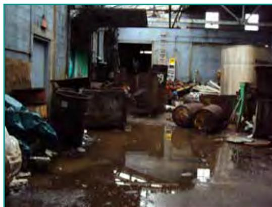
Example of a partially collapsed roof within a former manufacturing facility and the safety hazard posed by miscellaneous and unlabeled drums and containers of chemicals left in the building.
