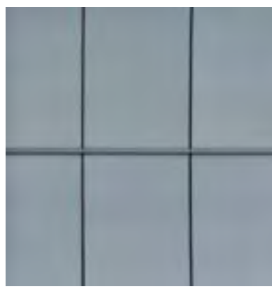
Back painted Glass - To match Existing. 17' OH, 5' Panels
