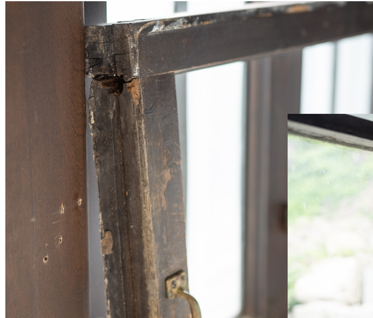
Detailed photo of the wood rot in original window
