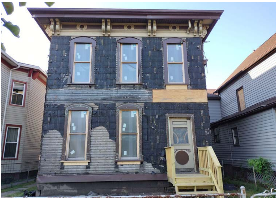
Documentation of 3401 Clinton post Transite siding removal 7/18/22
