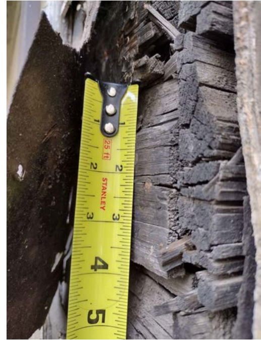
Documentation of existing layers of siding @ 3401 Clinton
