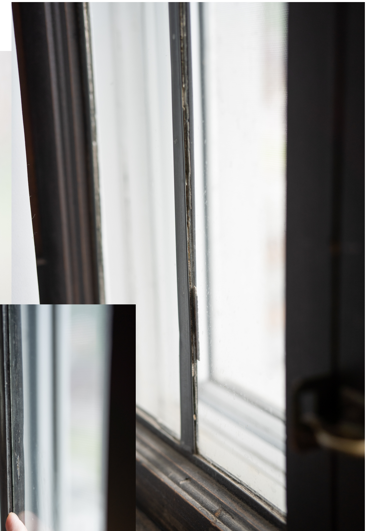
Disintegrating material in muntins
