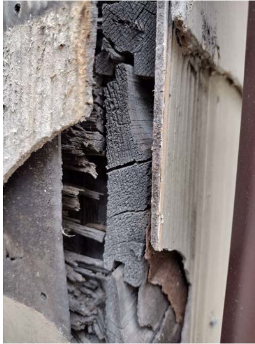
Documentation of existing layers of siding @ 3401 Clinton
