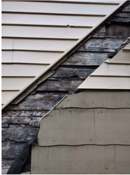
Vinyl siding over Asbestos Transite siding over Original old growth dutch lap
