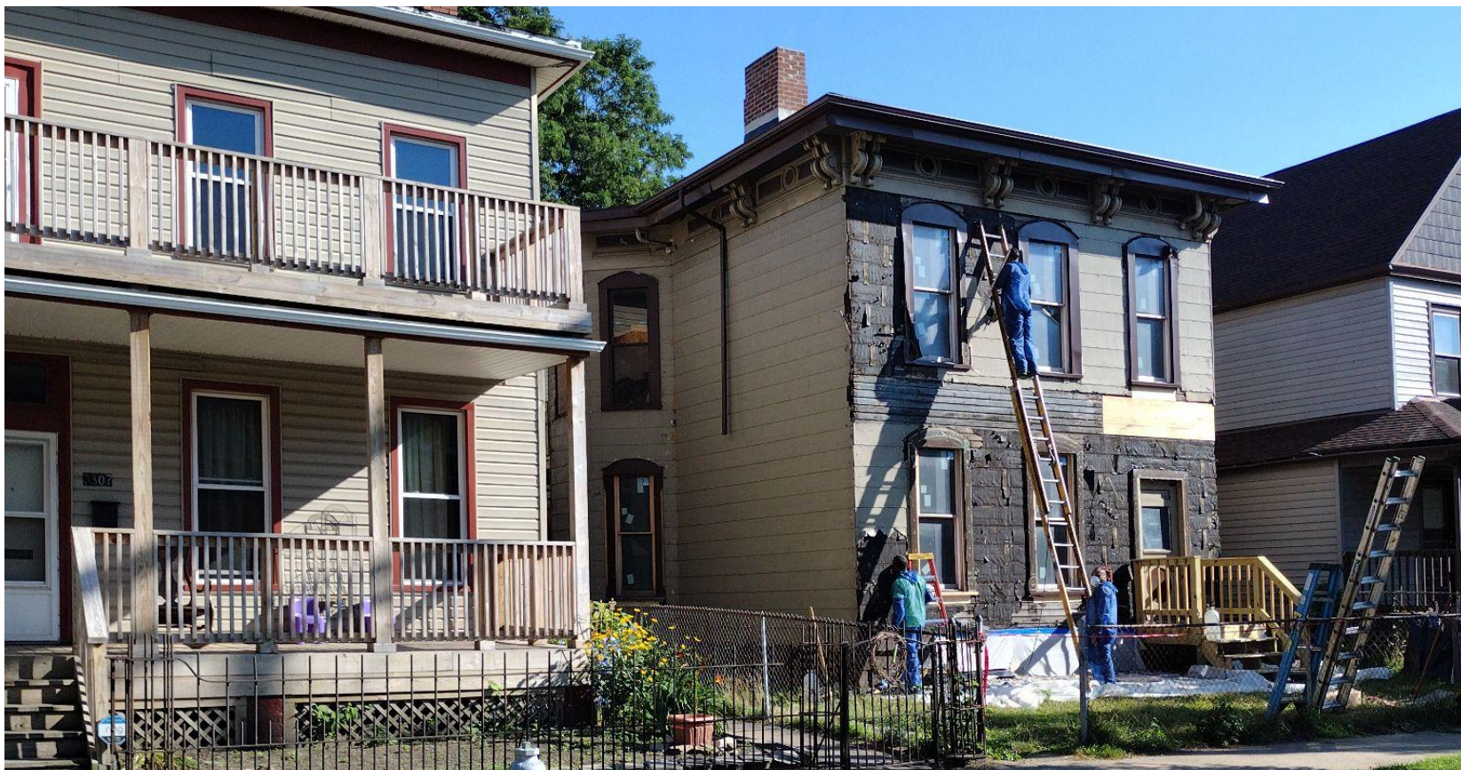
Asbestos remediation crew beginning work on 7/13/22
