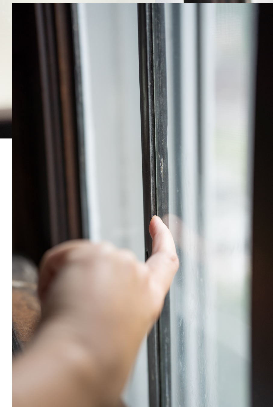
Large gap with no material holding in window pane
