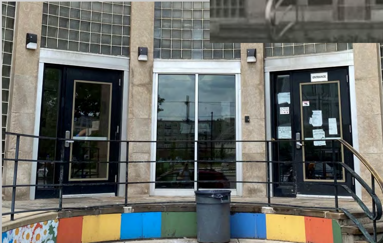
EXISTING CLEAR ANODIZED ALUMINUM ENTRY OPENINGS
