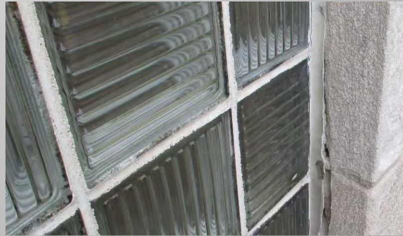
EXISTING GLASS BLOCK WITH 10 PARALLEL RIBS QUARTER TURN INSTALLATION – EXTERIOR VIEW
