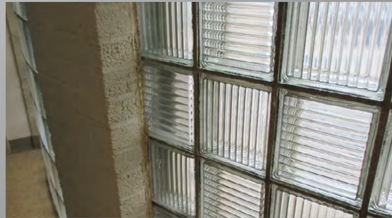
EXISTING GLASS BLOCK WITH 10 PARALLEL RIBS QUARTER TURN INSTALLATION – INTERIOR VIEW
