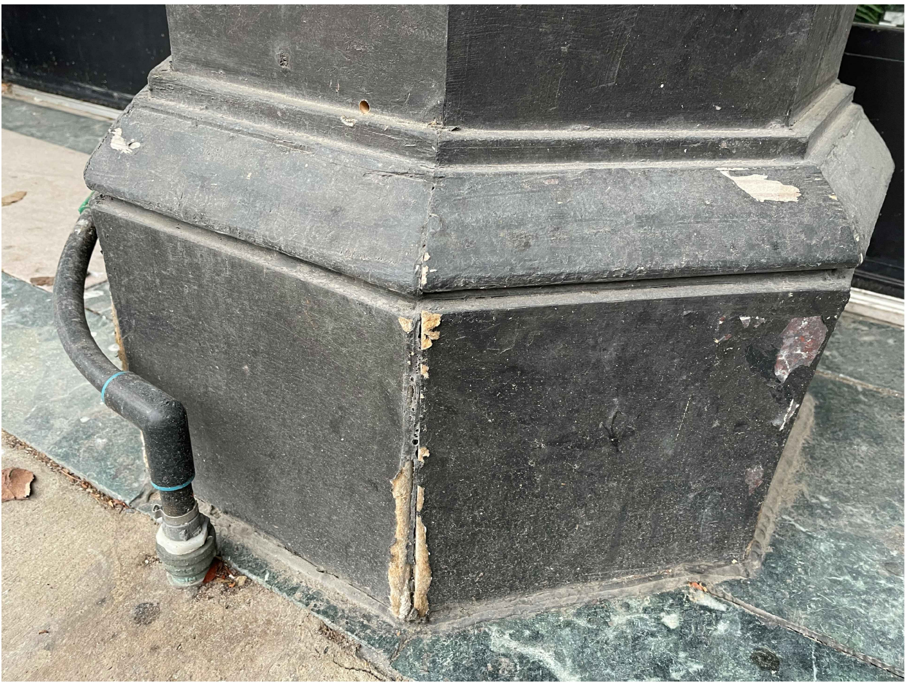
DETERIORATION AT EXISTING COLUMN BASES
