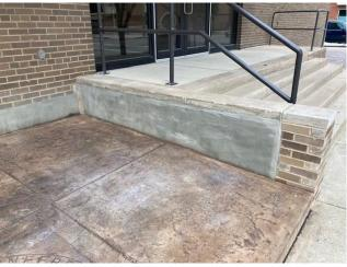
Stamped concrete and parging were added to seal area damaged and a planter space left in the center. It is a stone texture, stamped and was intended to color blend with the two sides of the building.
