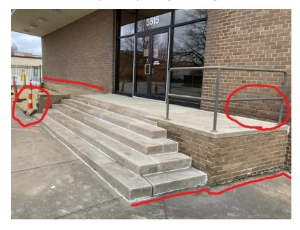
Area under soil line revealed parging on the surface of brick.
