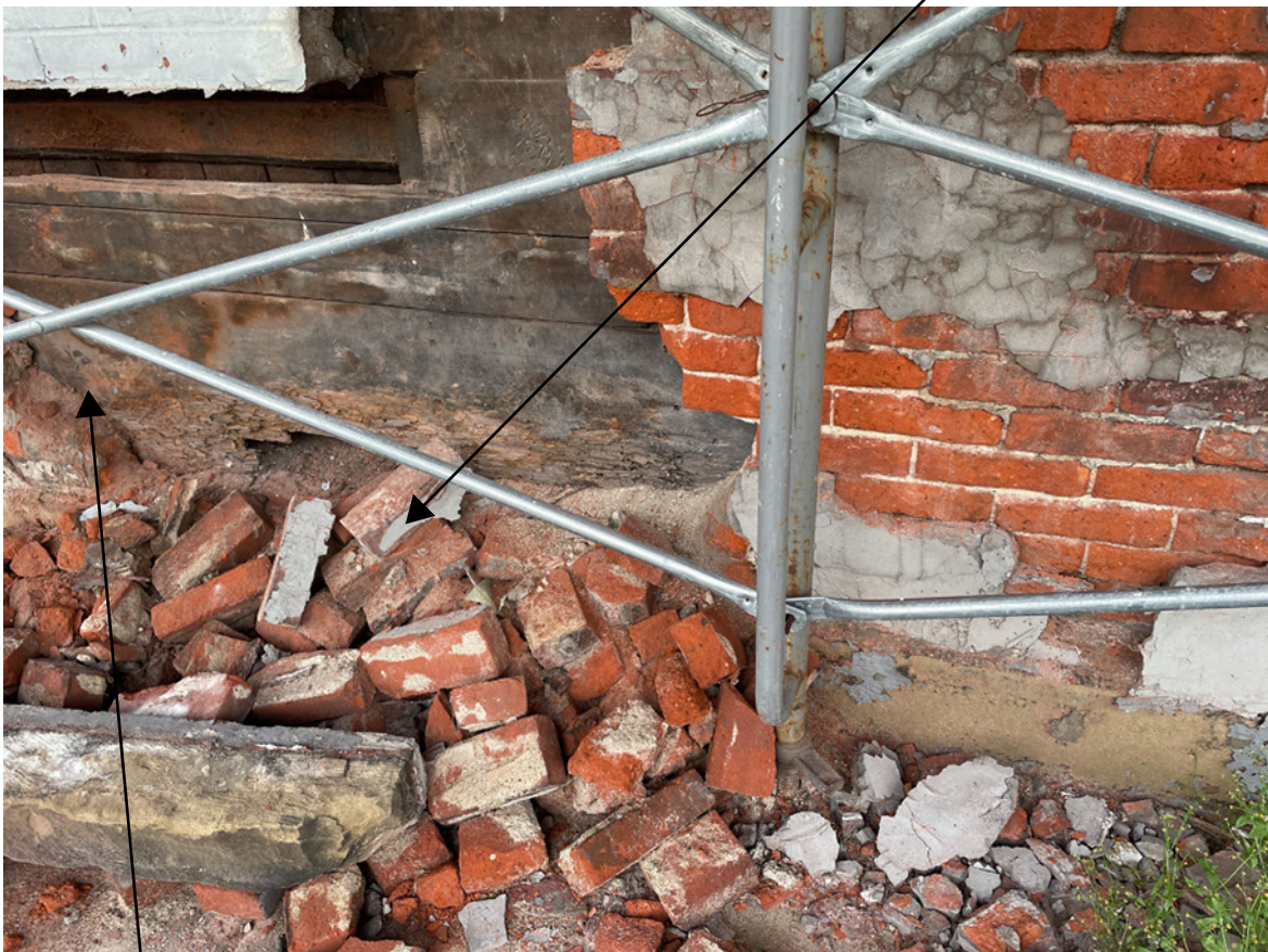
NO EXISTING TIES BETWEEN BRICK AND BUILDING WALL
