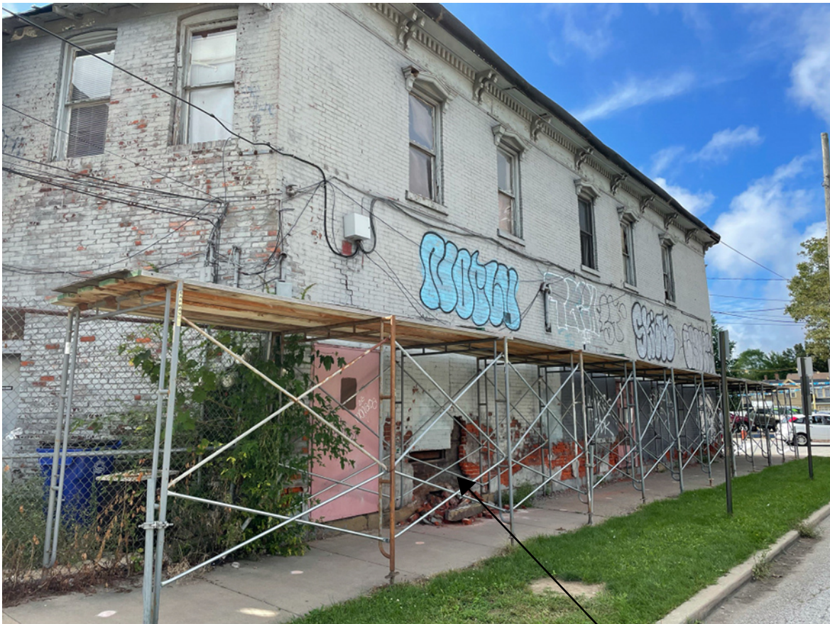
BRICK FAILED / FALLEN
