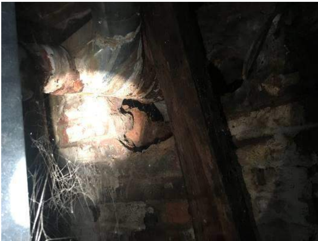
Broken main conduit in basement over panels
