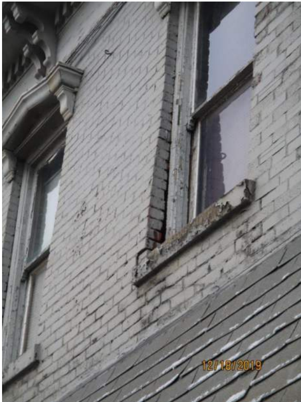
North exterior elevation brick veneer pushing out
