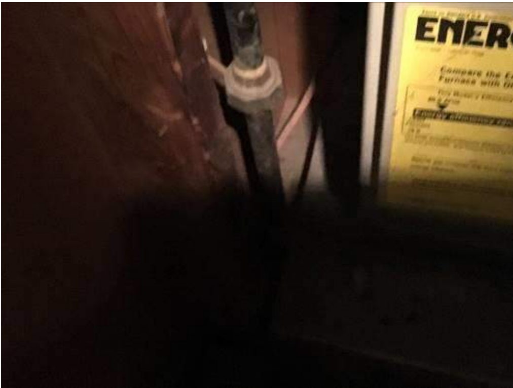
Pipe union in resident suite furnace plenum
