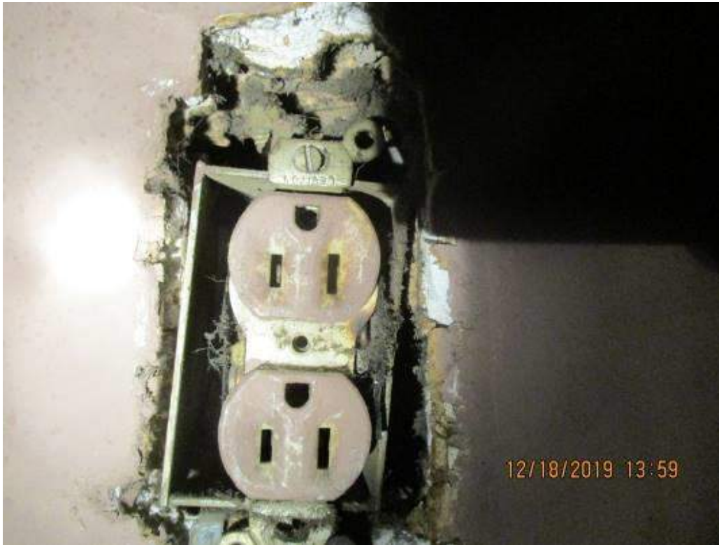
Deteriorated and ungrounded or questionably grounded receptacles
