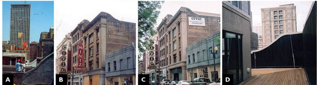
Figure 23. Colored flags marking the location of a proposed penthouse addition (a) were placed on the roof to help evaluate the impact and visibility of an addition planned for this historic furniture store (b). Based on this evaluation, the addition was constructed as proposed. It is minimally visible and compatible with the 1912 structure (c). The tall parapet wall conceals the addition from the street below (d).
