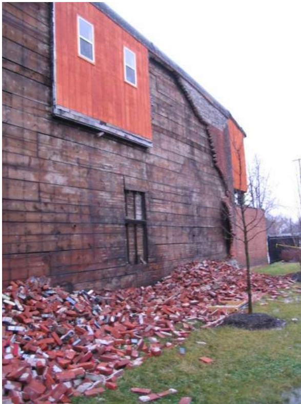
West elevation prior brick veneer collapse
