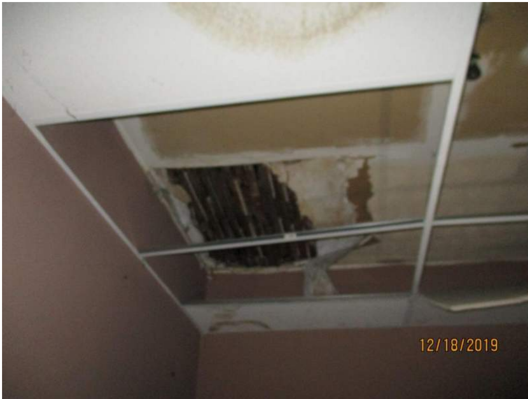
Minor water damage to roof framing and plaster finishes
