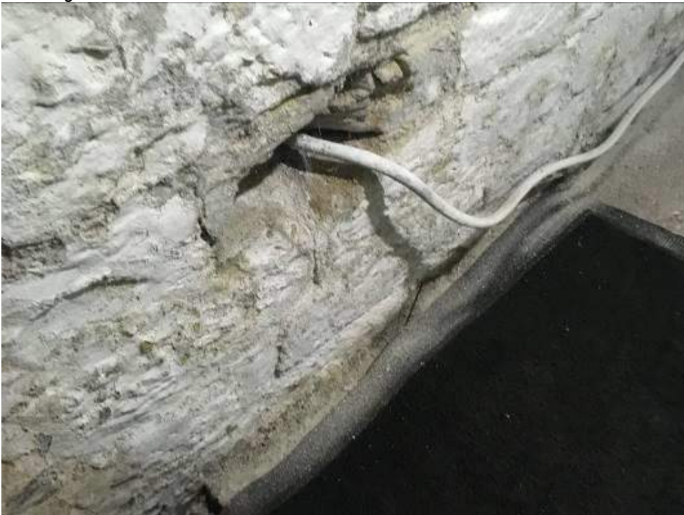
1", undersized water entry
