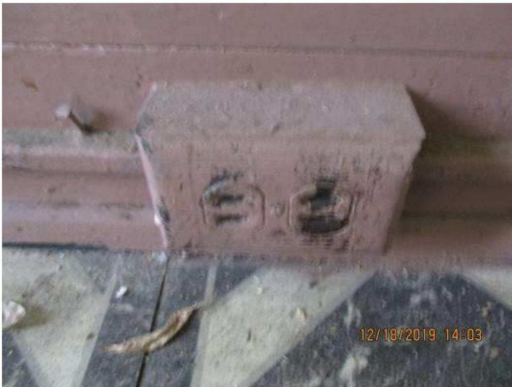
Deteriorated and ungrounded or questionably grounded receptacles
