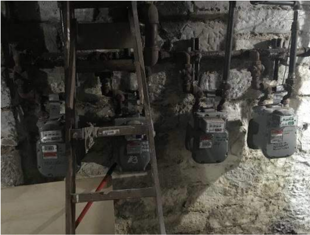
Rusted gas manifold
