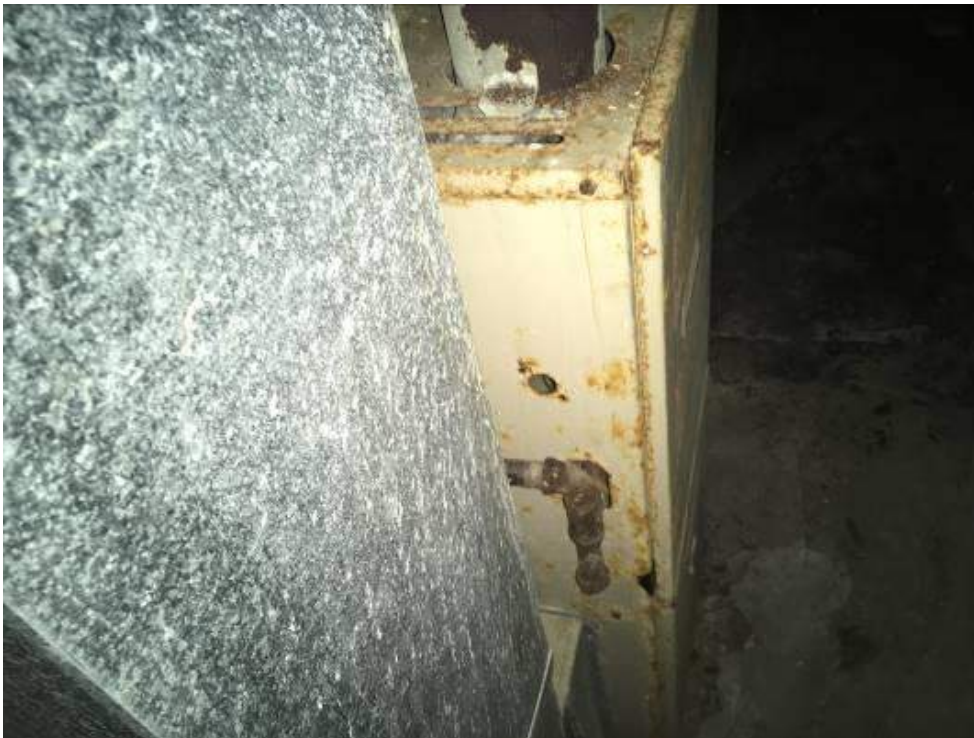
Rusted furnaces and flues in basement
