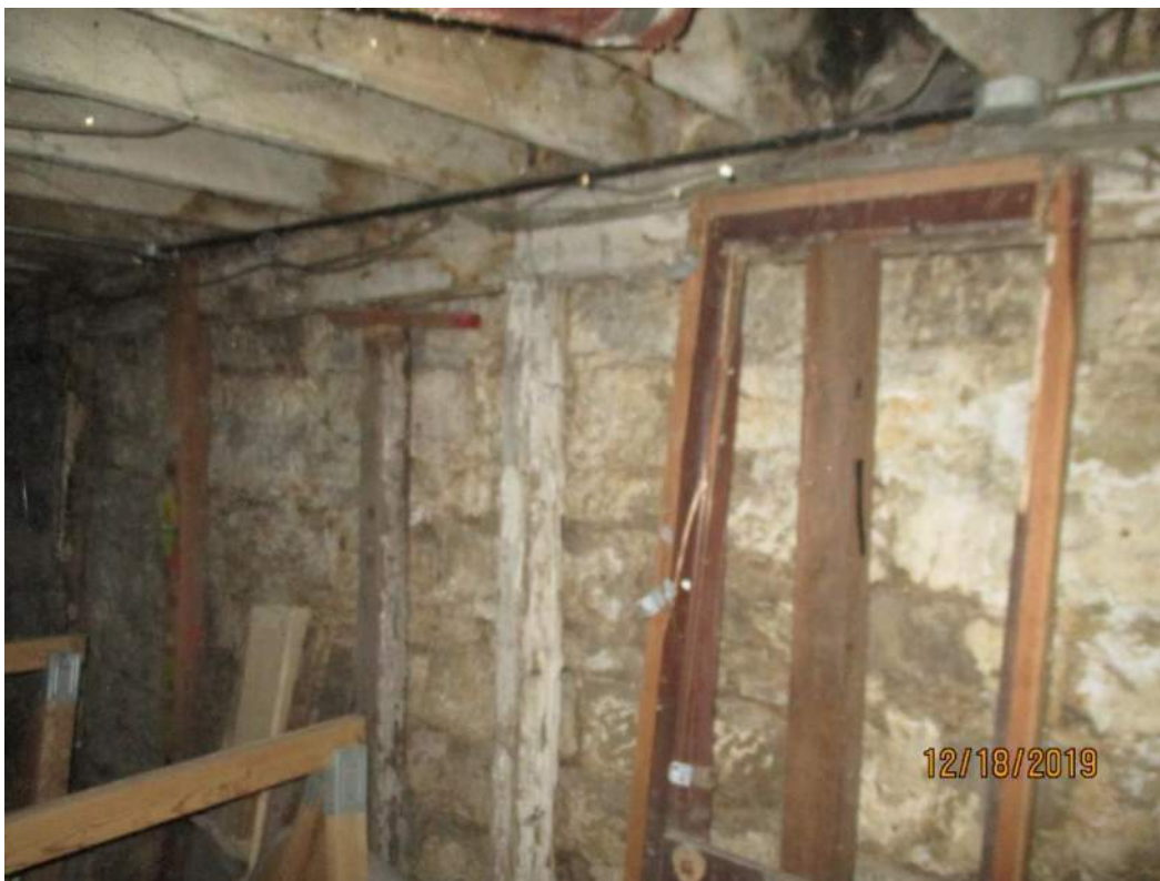
Existing 4x girder line supporting first floor framing independently of the basement stone wall
