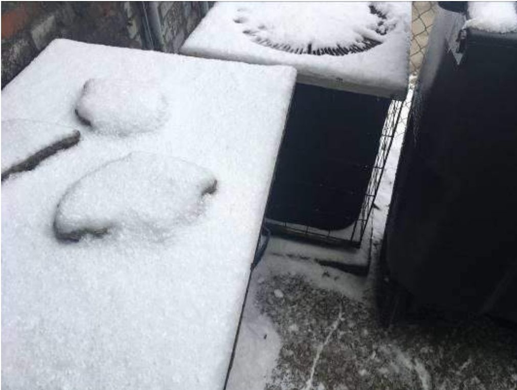
AC condensing unit on grade
