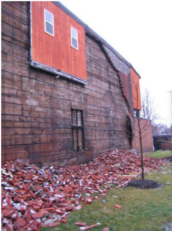
West elevation prior brick veneer collapse
