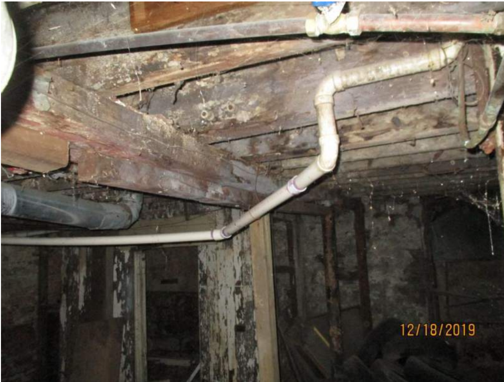
Existing 4x10 girder beam line with post removed and floor sagging approx. -2"
