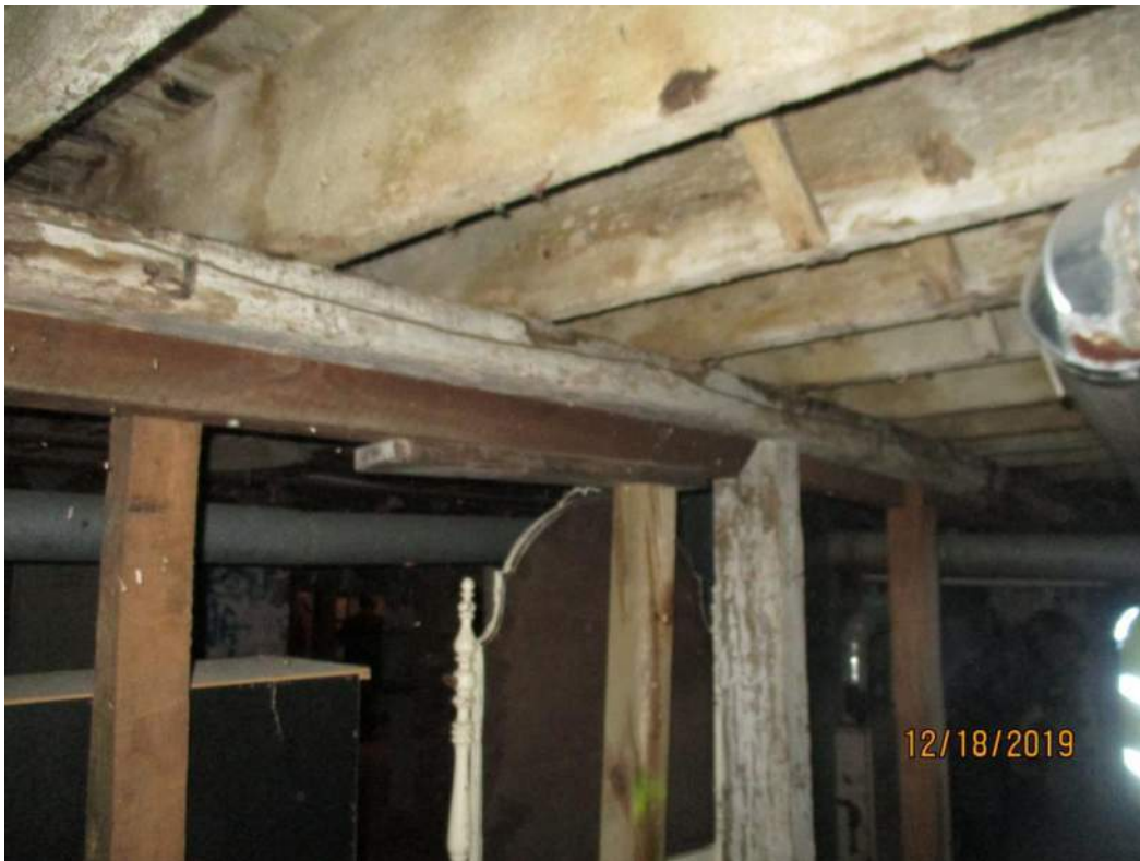
Existing girder beam line subdividing basement
