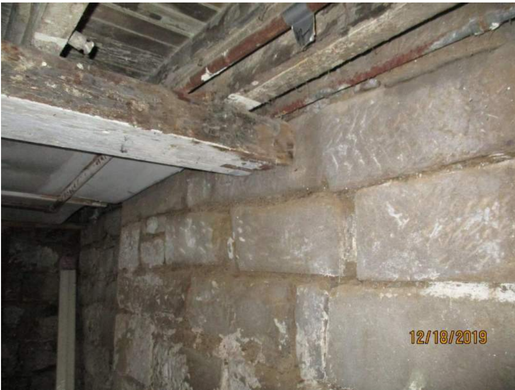
Existing 4x10 girder beam not supported by wall and no wood post in place
