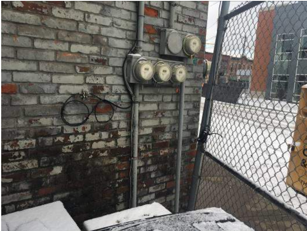
Electrical service metering
