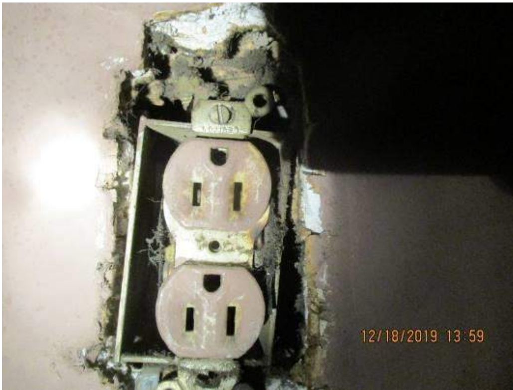
Deteriorated and ungrounded or questionably grounded receptacles
