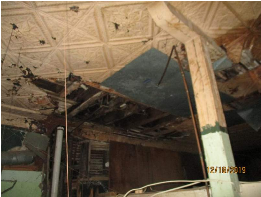
Water damage to second and first floor framing due to second floor bathroom
