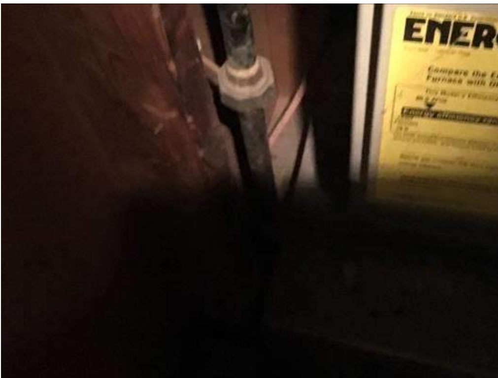
Pipe union in resident suite furnace plenum
