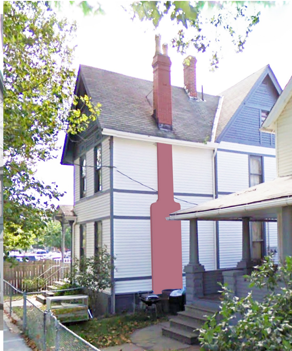
North elevation: Note the demolition of the decorative Victorian brick chimneys including terra cotta chimney-pots. What remains of externally expressed brick chimney no longer makes any visual sense. (brick color added)
