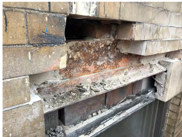
STEEL CHANNEL AND ANGLE @ WINDOW HEAD
