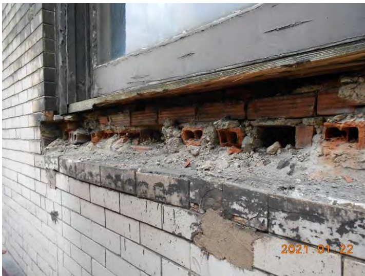
MULTI-WYTHER BRICK MASONRY BELOW 2ND FLOOR WINDOW SILL
