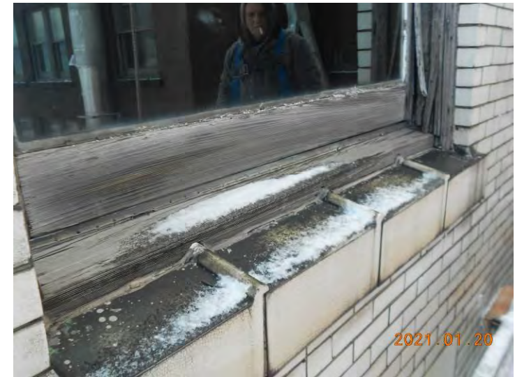
ROTTED, CRACKED, AND FAILED WOOD WINDOW FRAME
