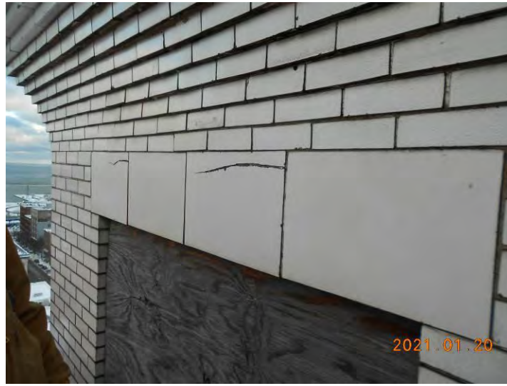
CRACKED TERRA COTTA WINDOW HEAD @ STEEL BEARING ANGLE
