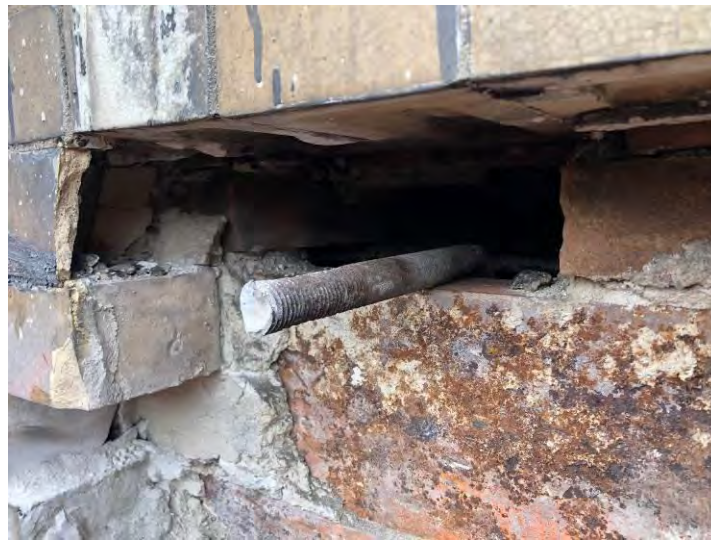
TYPICAL EMBEDDED J-BOLT FROM PREVIOUS FIRE ESCAPE
