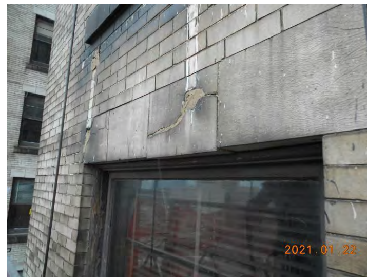
CRACKED TERRA COTTA WINDOW HEAD @ STEEL BEARING ANGLE
