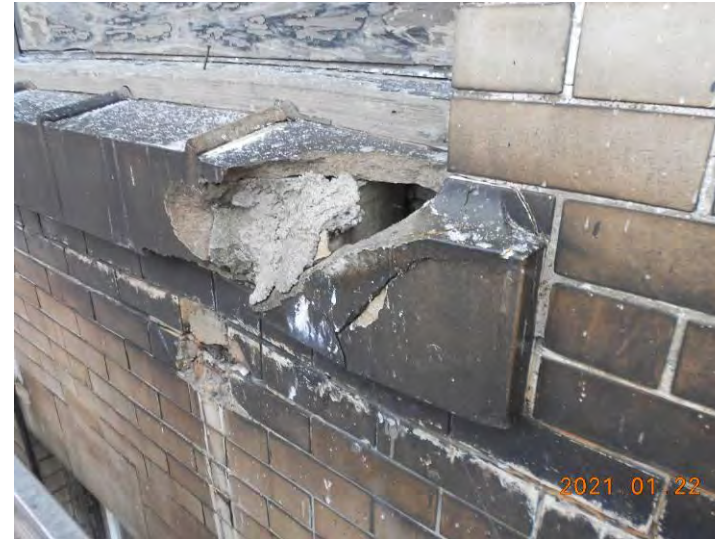
CRACKED AND SPALLED TERRA COTTA UNIT @ WINDOW SILL
