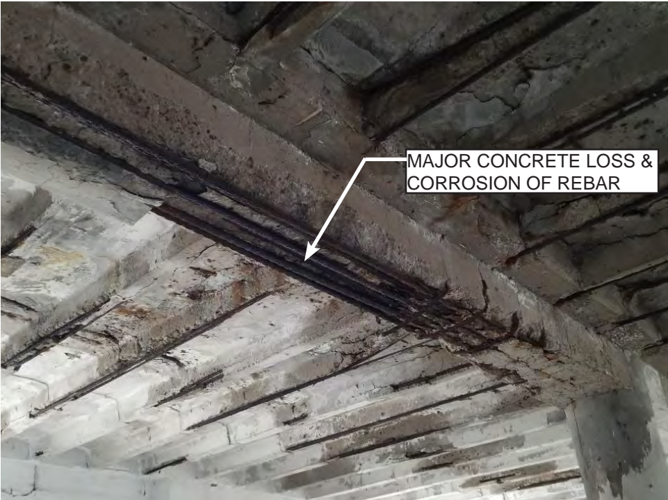
CONDITION OF EXISTING BEAMS
