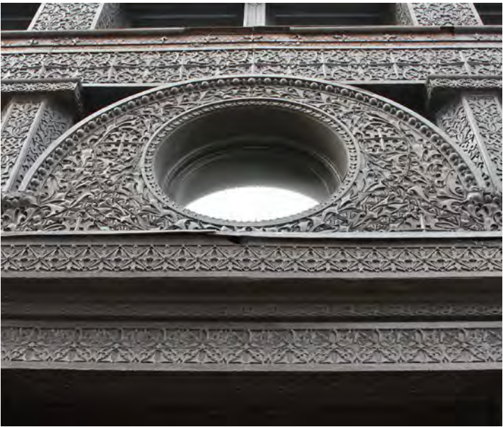
DETAIL OF CAST IRON @ 2ND FLOOR
