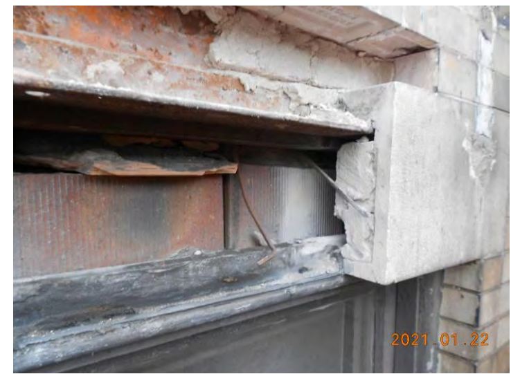
STEEL BEARING ANGLE AND TERRA COTTA HOOK @ WINDOW HEAD
