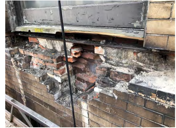
PLATE @ 5TH FLOOR WINDOW SILL WITH STEEL ANGLE
