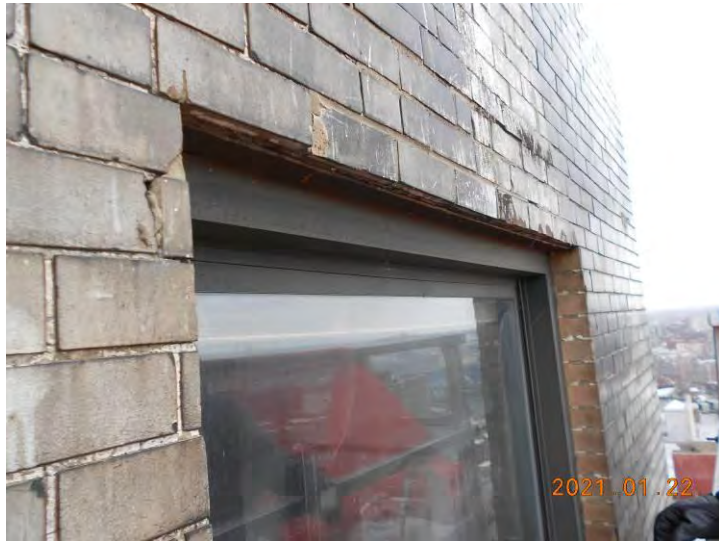
ADDED OPENINGS, WINDOWS, AND LOOSE LINTELS
