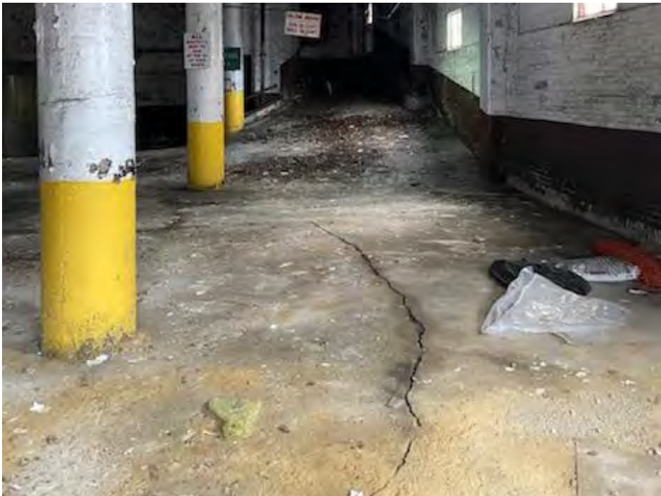
CONDITION OF EXISTING SLAB ON GRADE
