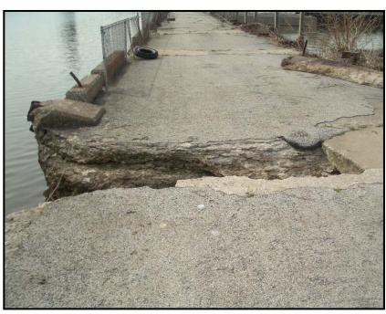
Pier must be rebuilt along entire length.
