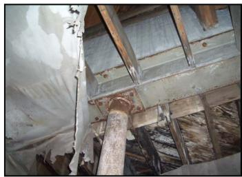
Second floor wood joist and wood sheathing has completely deteriorated.
