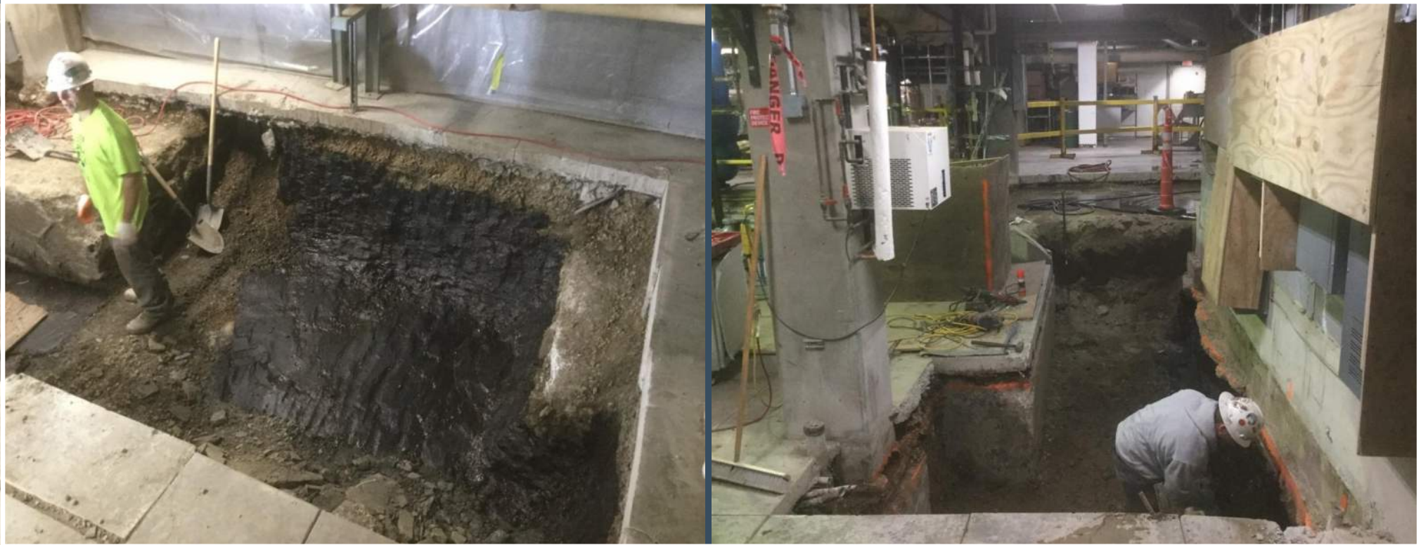
EXCAVATION REQUIRED TO MITIGATE THE CIRCUMSTANCES OF THE EXPANSIVE SHALE FROM EXISTING BASEMENT.
