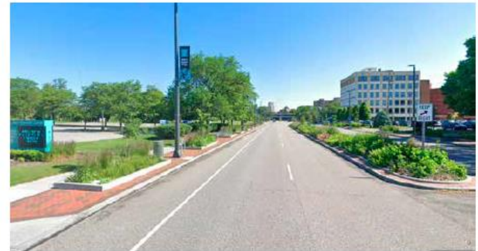
6 | VIEW FROM EAST 22ND STREET LOOKING NORTH
