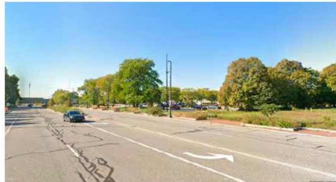
5 | VIEW FROM EAST 22ND STREET LOOKING SOUTH
