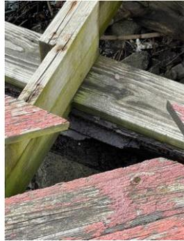
EXISTING WOOD DECKING TO BE REMOVED. STEEL BEAMS AND FOOTINGS TO REMAIN.
