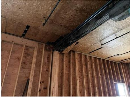
WEST FACADE INTERIOR - NEW CONSTRUCTION TO BE REMOVED IN ENTIRETY. ALL HISTORICAL ELEMENTS: STRUCTURE, DECK, CEILINGS AND FLOORS TO REMAIN.
