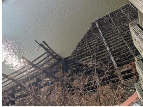
EXISTING WOOD DECKING TO BE REMOVED. STEEL BEAMS AND FOOTINGS TO REMAIN.
