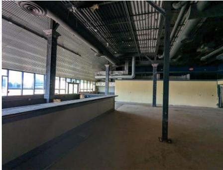
INTERIORELEMENTS AND STRUCTURE - TO BE REMOVED IN ENTIRETY
