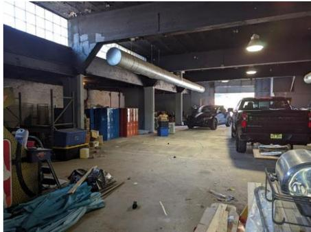
NON-LOADBEARING WALLS - TO BE REMOVED IN ENTIRETY CONCRETE STRUCTURE - TO REMAIN
