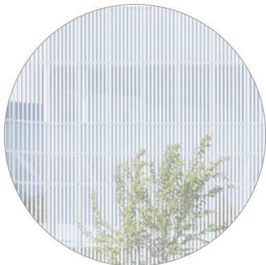
SSG _ INSULATED GLAZING UNIT WITH LOW-E COATING AND CUSTOM FRIT PATTERN
