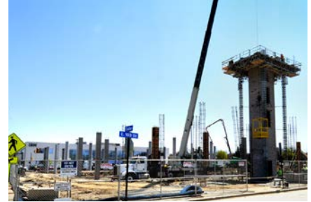
New Meijer Grocery Store Under Construction
