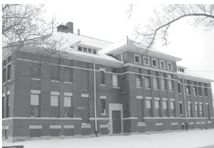
Former Willard Elementary
