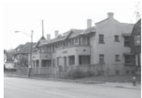
Historic apartment block on Miles Avenue
