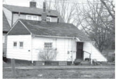
700 square foot house on Reno Avenue
