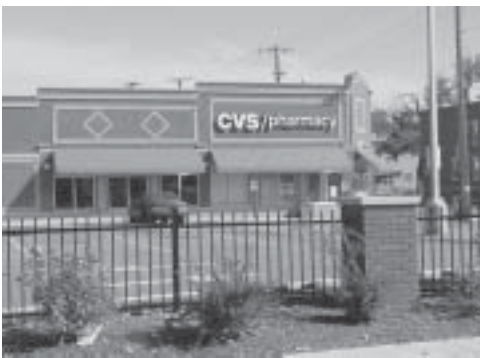
CVS on Cleveland's west side: a rigorous design review process resulted in a building that is very compatible with its surroundings.
