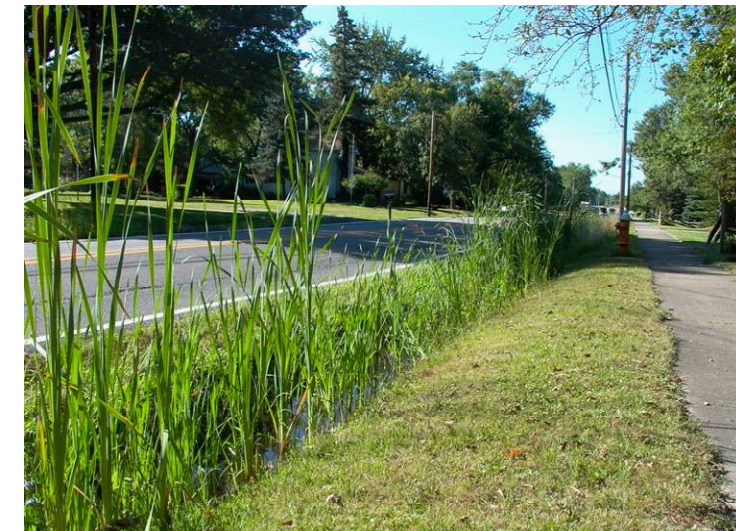
Swale along residential street
