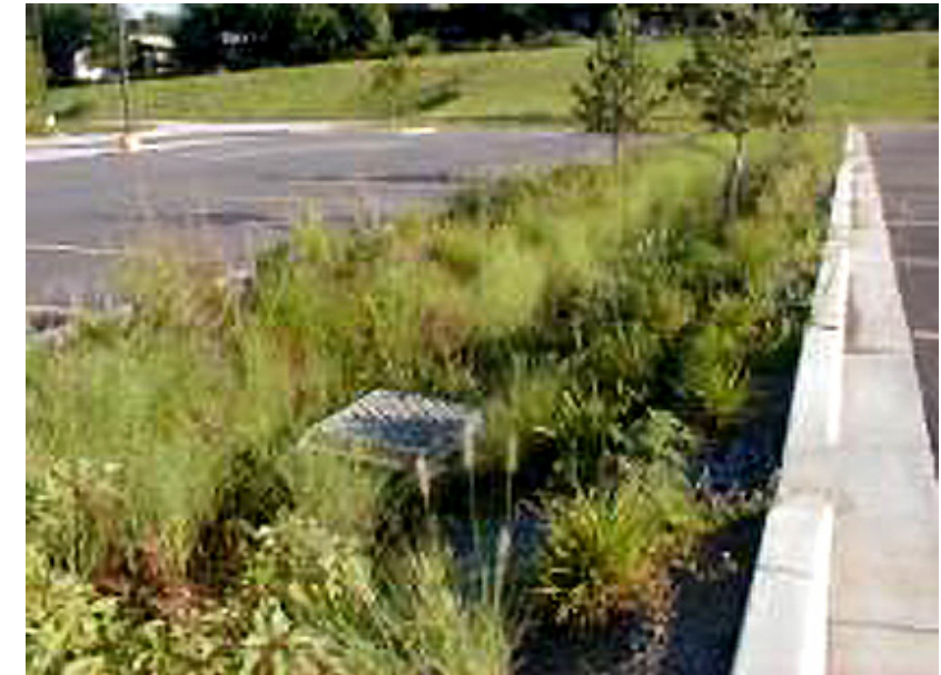
Parking lot vegetated swale
