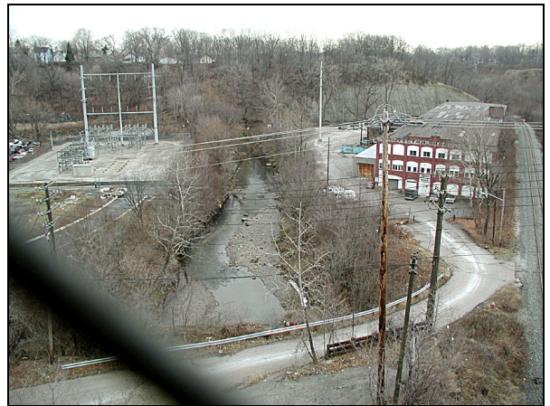
Industrial Facility below US-42
