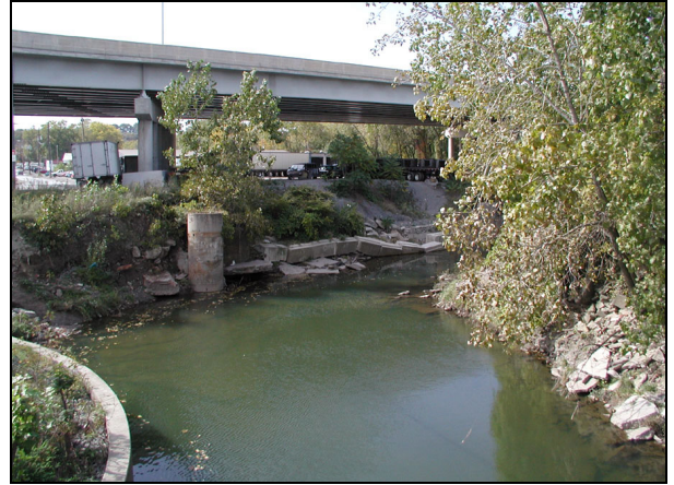
Parking of Truck Rigs under Jennings Freeway
