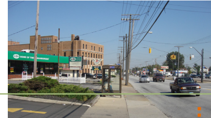
Bus Shelters Encroach Sidewalk Area
