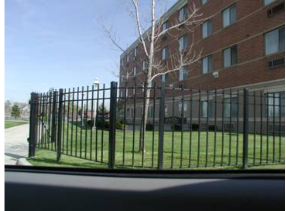
Natural access control is a technique commonly used by planners and designers to create a strong perception of safety in the physical environment.
