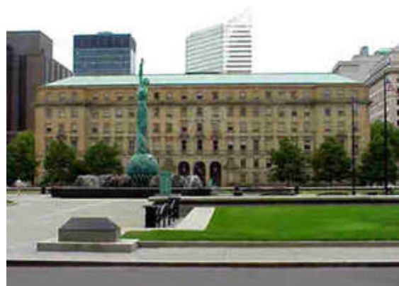
CMSD Administration Building located in downtown Cleveland is the headquarters of the Cleveland Public Schools
