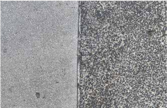
ENHANCED CONCRETE 1 AND 2 COLORED CONCRETE WITH SPECIAL FINISH AND AGGREGATE PROPOSED FINISH IS TOPCAST (SIMILAR TO SANDBLAST)
