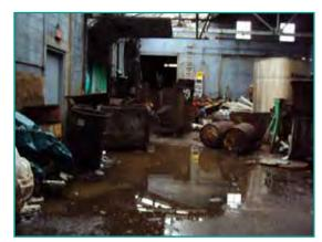
Example of a partially collapsed roof within a former manufacturing facility and the safety hazard posed by miscellaneous and unlabeled drums and containers of chemicals left in the building.
